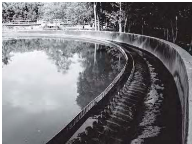
Fig. 18.5 Water clarifier
