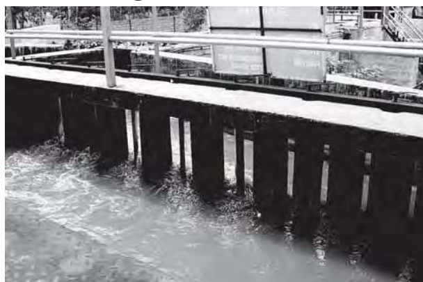
Fig. 18.4 Grit and sand removal tank
